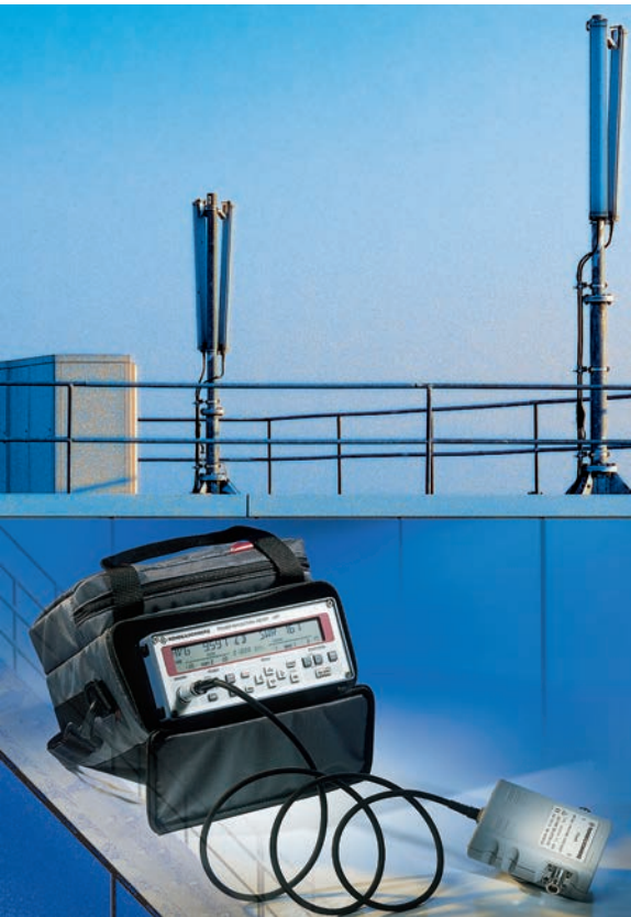
The R&S® NRT is also ideal for mobile use, e.g. for measurements on GSM antennas
